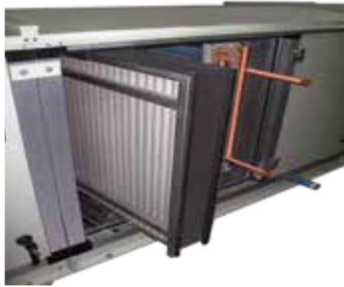
Figure 5: Eliminators installed on rails are removed from cleaning.
