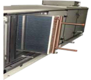
Figure 4: Coils are installed on rails and are free to be removed from the AHU for cleaning.
